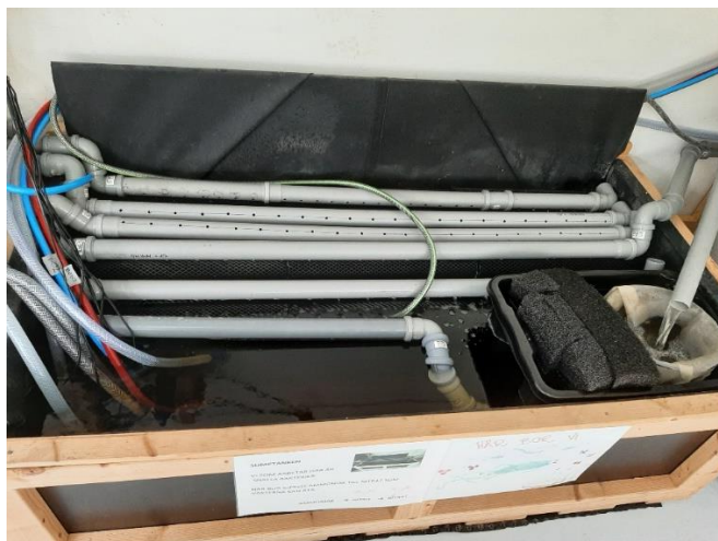
Fig. 7 – The sump tank in the demo at Campus Roslagen has the main purpose to provide a volume buffer: If water level variations happened in the fish tank this would stress the fish. In this case the sump is also used to have the biofilter and the mechanical filter.
