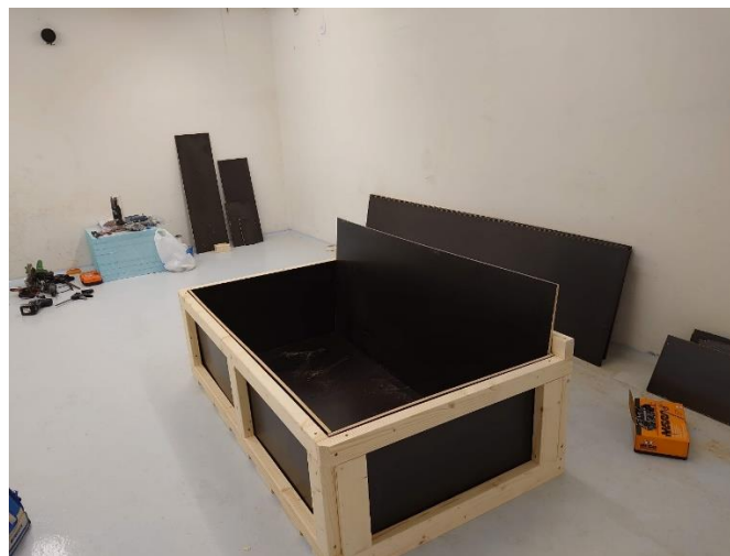
Figure 6 - Sump tank during construction, the inside of the tank was later coated with a rubber sheeting.
