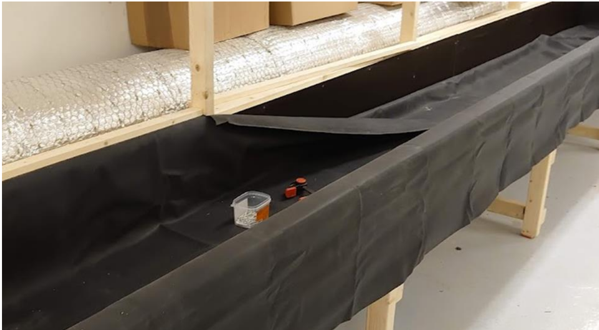
Figure 2. Rubber liner fastened in DWC
