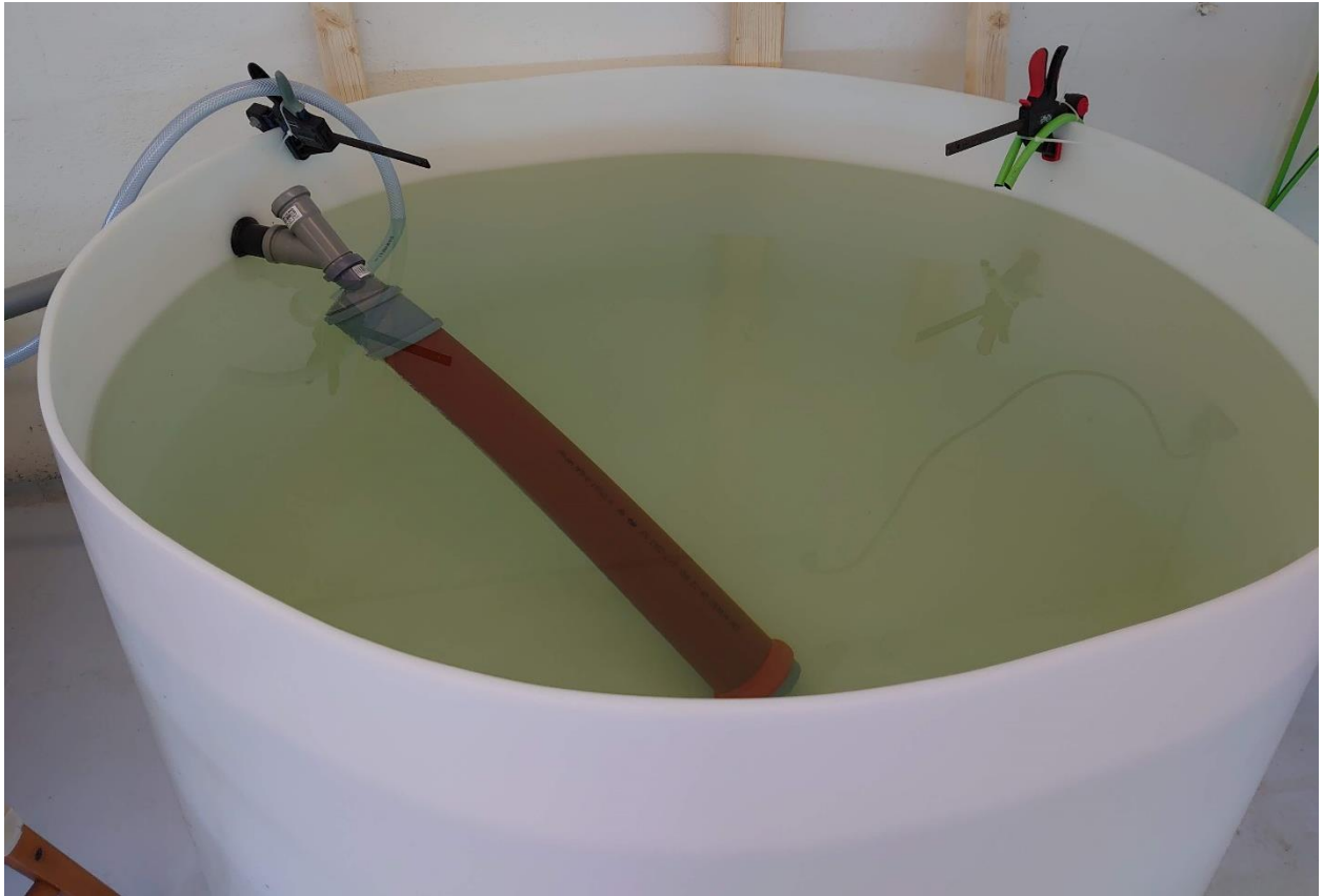
Figure 6. Fish tank during construction. Water exits the tank from the bottom of the tank, by rising through the red pipe, the grey Y-pipe, the black pre-welded outlet and back to the sump. The inlet water hose in the picture is a very temporary setup during construction and should not be considered a recommendable installation.
