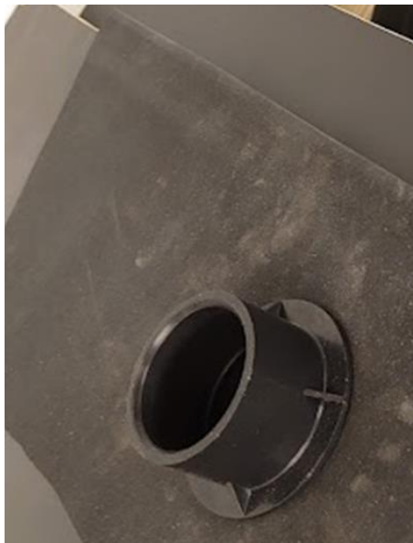
Figure 4. outlet fitting through rubber lining
