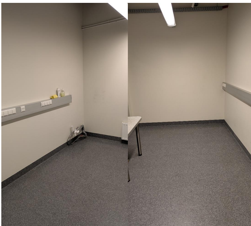
Figure 1. Room prior the demonstration unit construction.
