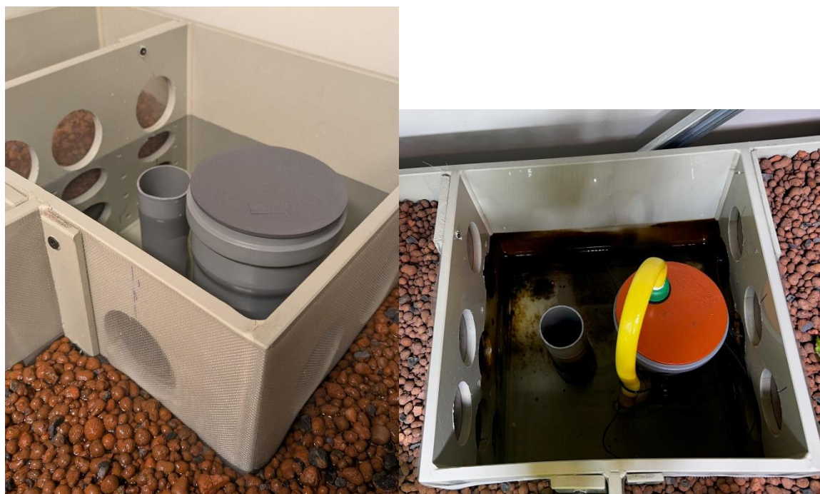
Figure 5. Initial siphon design (left) and the final, functioning siphon with fill up time of 10 minutes and bed emptying time of 45 sec.
