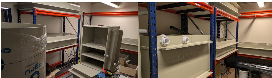
Figure 4. Modifying of containers to allow proper fitting within the shelving structure, and preparing overflow fittings.
