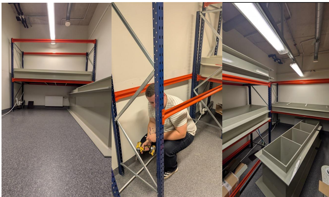
Figure 3. Mounting supporting framework, and mounting the main system components.
