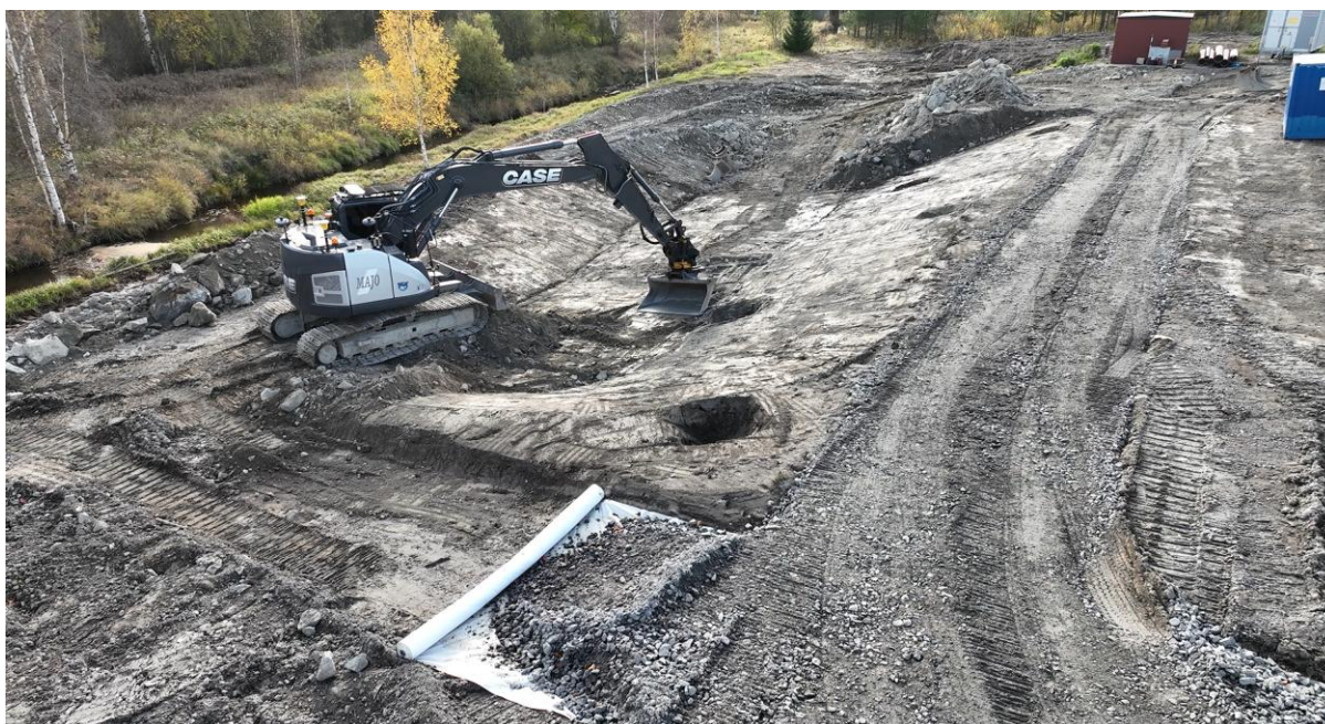
Porten pilot site during construction in October 2025.
