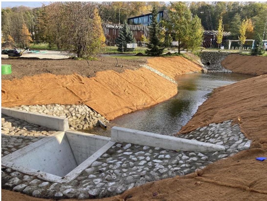
View from the outflow of the designed sedimentation and detention pond.
