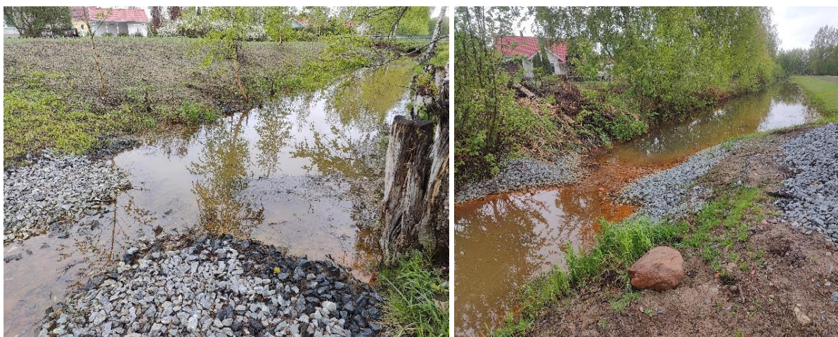
The wetland pilot solution features two different types of filtration dams. The first photo shows the biochar and gravel dam, and the second photo shows the limestone and pumice stone dam.
