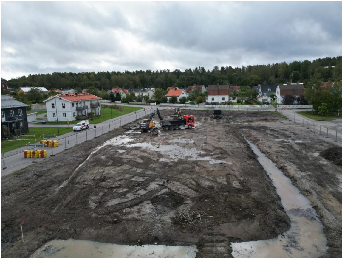
Construction works in Broberg in September 2025.
