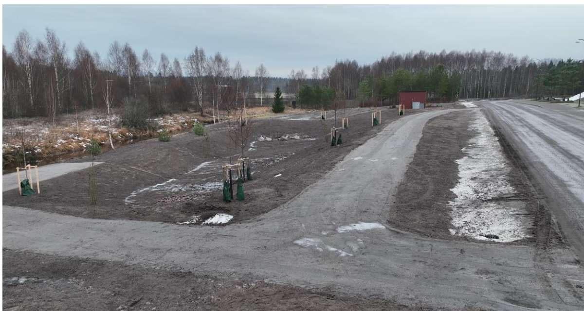
Completed pilot site in December 2025.
