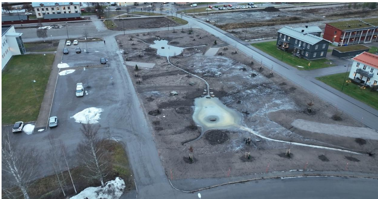
Completed pilot site in December 2025. Green area B is shown in the forefront.
