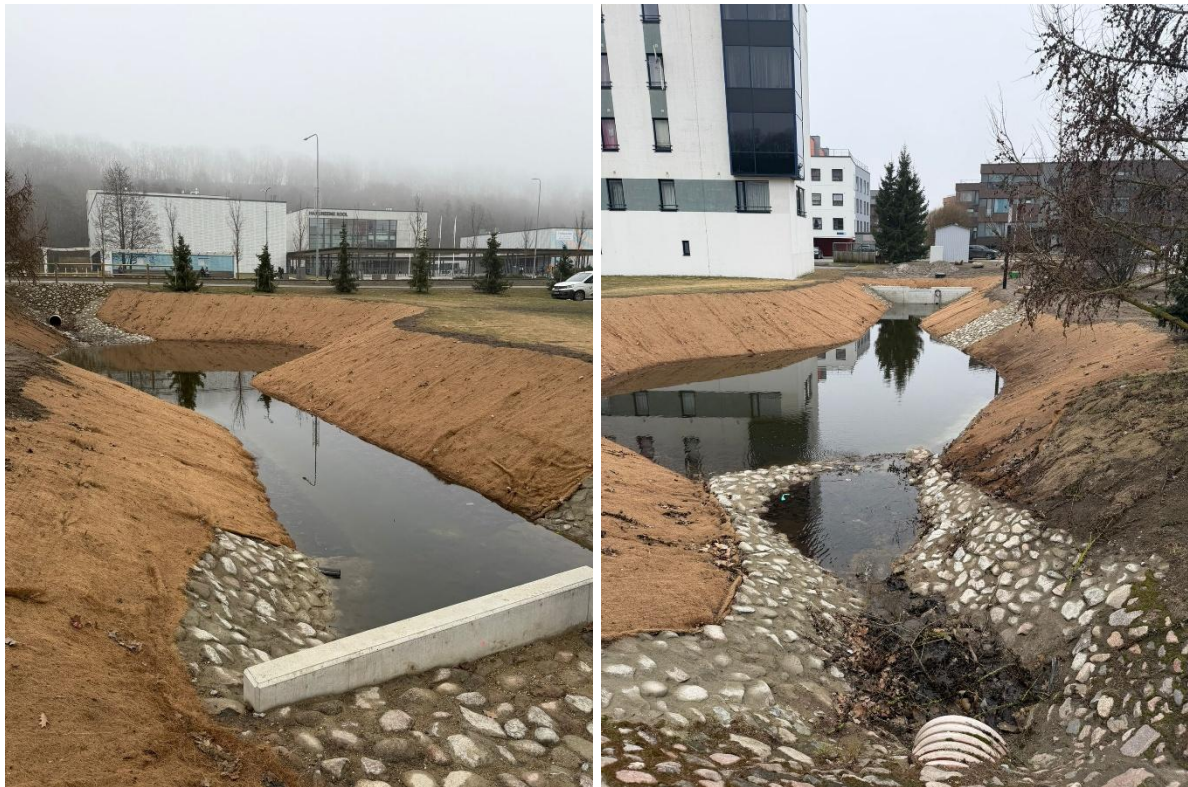
The completed retention pond.
