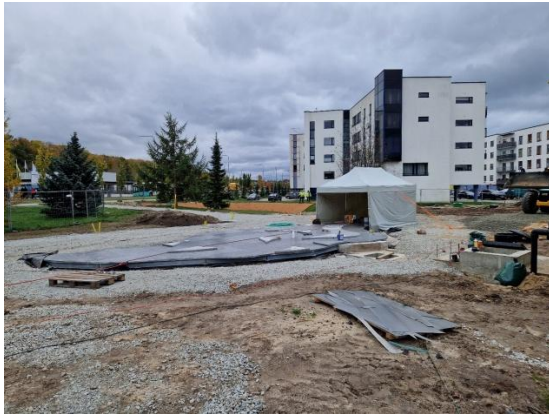
Construction of the above-ground part of the fountain.
