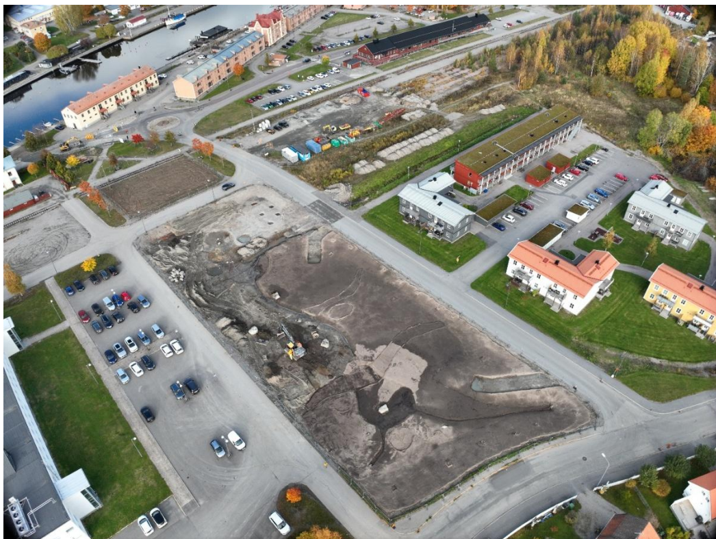
Construction works during October 2025. Green area B is in the forefront.
