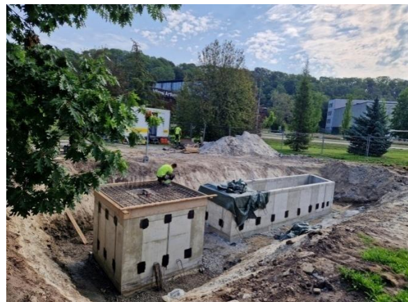
Underground chambers of the designed fountain.
