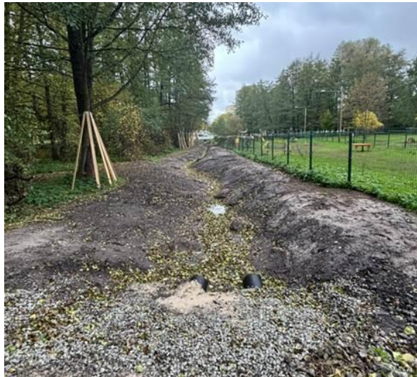
Downstream view of the drain ditch.
