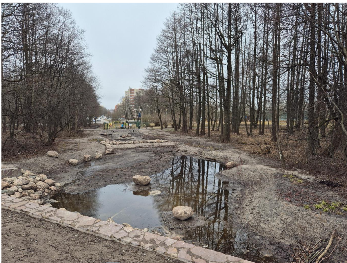
The first retention pond.
