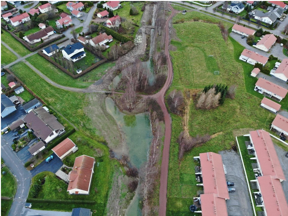
Wetland after construction. Due to the dams, the wetland now has a permanently higher water level.
