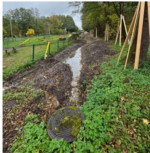
Upstream view of the drain ditch.
