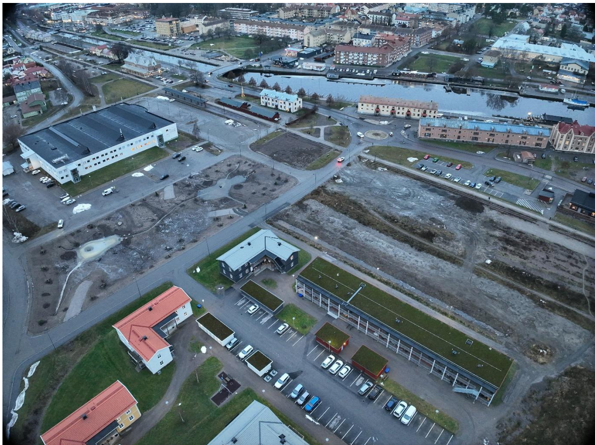
Completed pilot site in December 2025.
