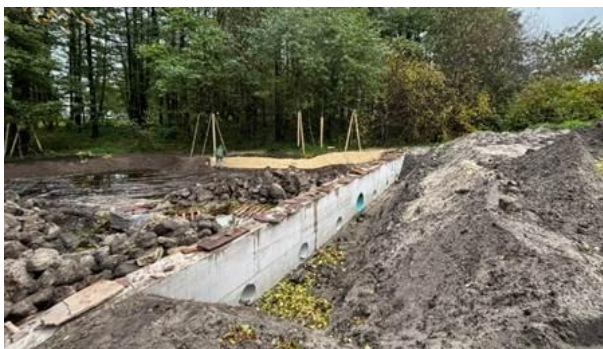
First pond connection with the pipes from the Tammsaare Road.
