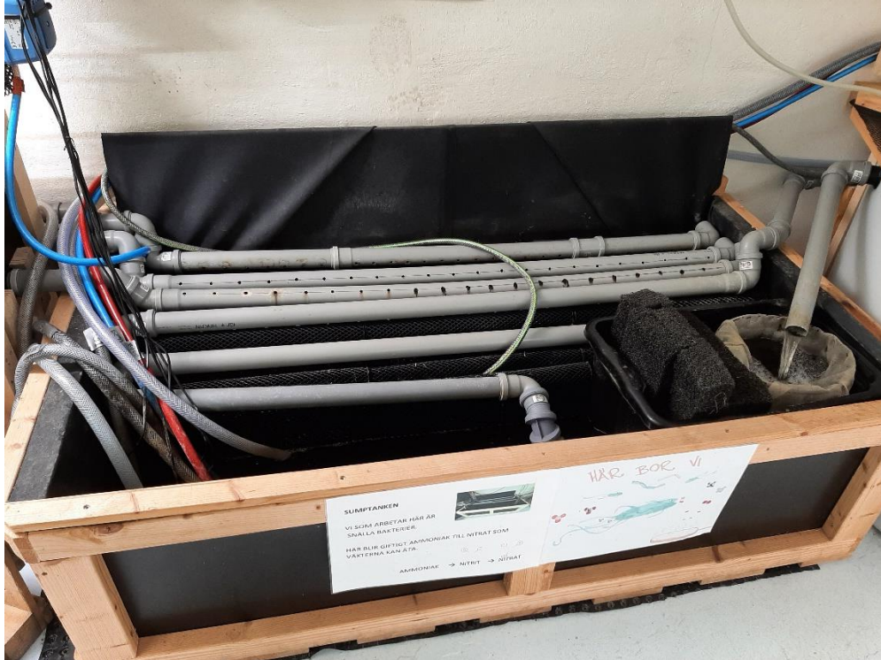
Figure 7. Biofilter for an aquaponics system at Campus Roslagen, Norrtälje.
