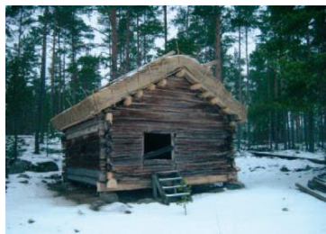
Restored reed roof of a barn. Rymättylä, Southwest Finland. Photo: Markku Hyvönen
