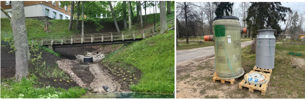
Figure 4.4. Stormwater management site in Smiltene and the tanks before installation.
