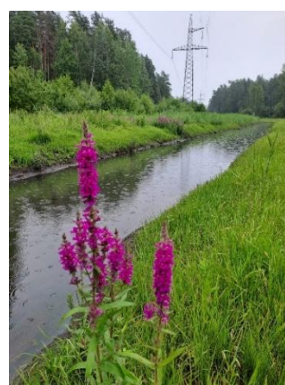
Figures 38. Šmerļupīte Pilot Site after construction
